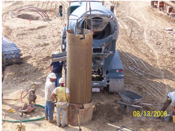
Figure 7: Drilling and placing caissons.
