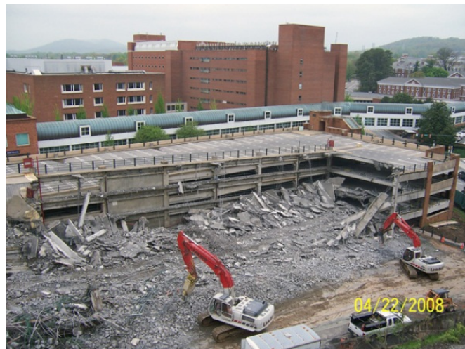
Figure 3: Demolition of the existing parking garage.
